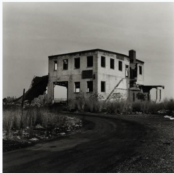
Abandoned Building, Caven Point, N.J. 1984
